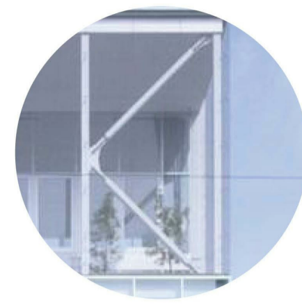
B- WHITE STEEL STRUCTURE
