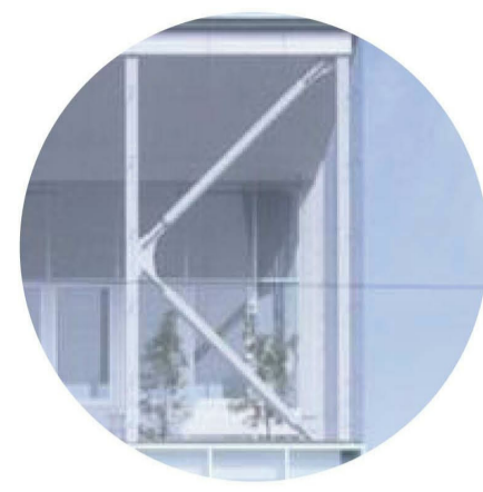
B- WHITE STEEL STRUCTURE
