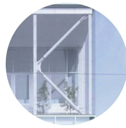
B- WHITE STEEL STRUCTURE
