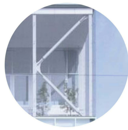
B- WHITE STEEL STRUCTURE
